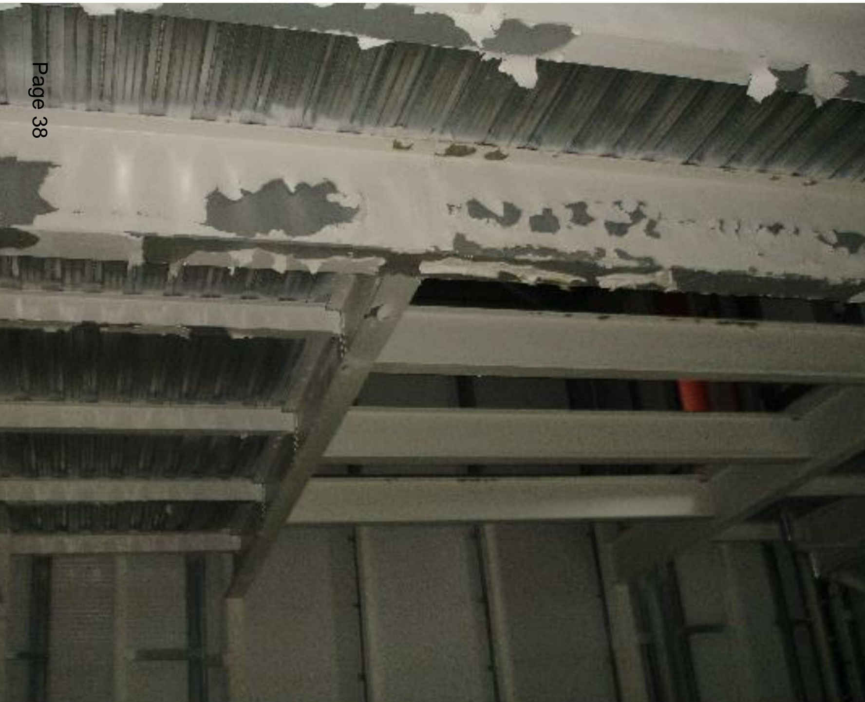
Defective paintwork on interior steel frame
